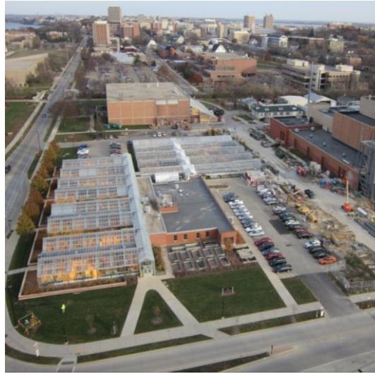
Walnut Street Greenhouses
